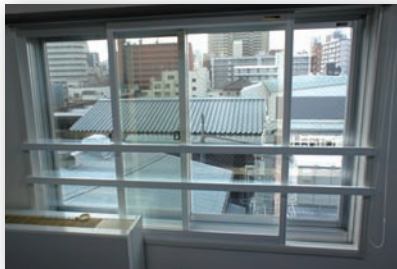
Double-pane windows at the Head Office
