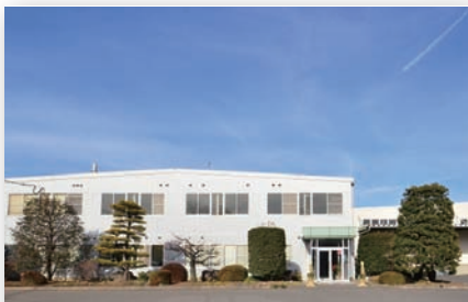
Dec. ... Made Suda Shoji, Inc. a consolidated subsidiary
